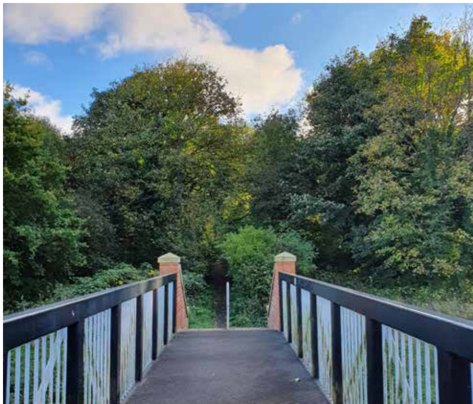
Bridge over Chesterfield Canal at the north canal link.
