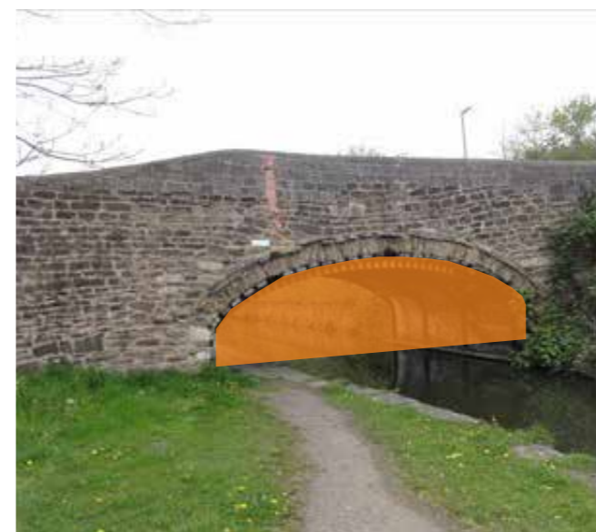
Mill Green Bridge, over Chesterfield Canal
