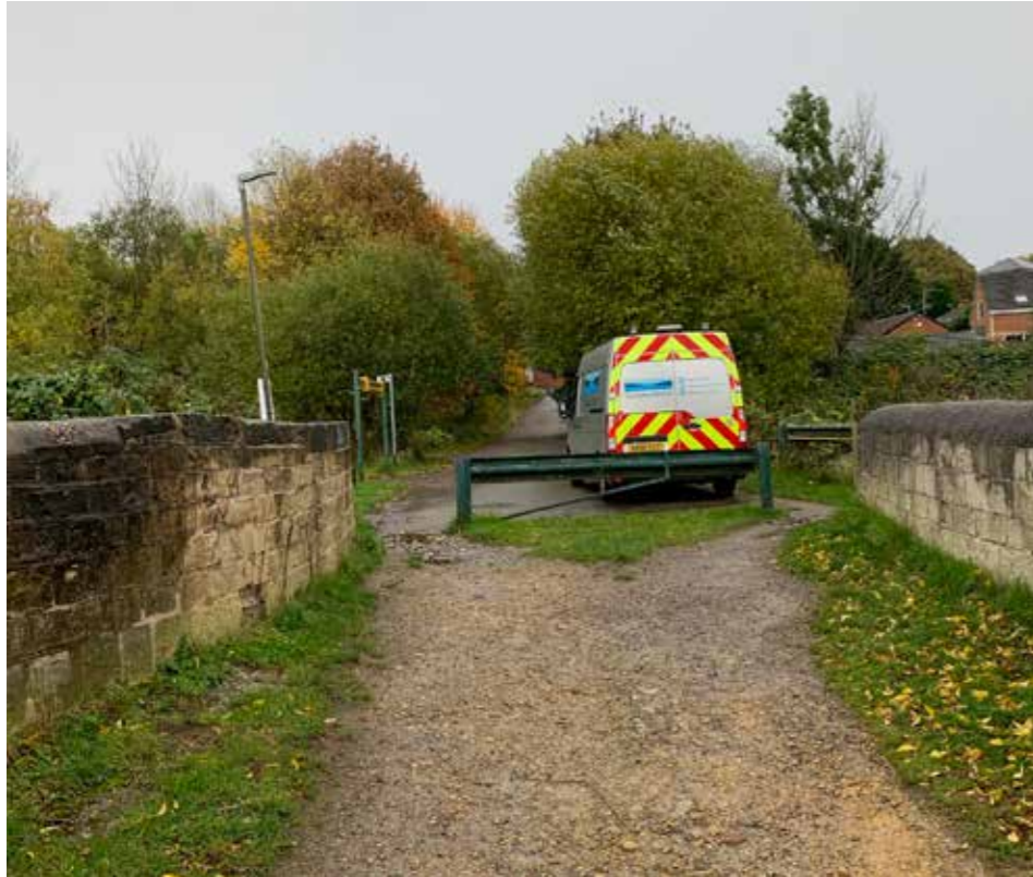
Mill Green bridge over Chesterfield Canal at the south canal link.
