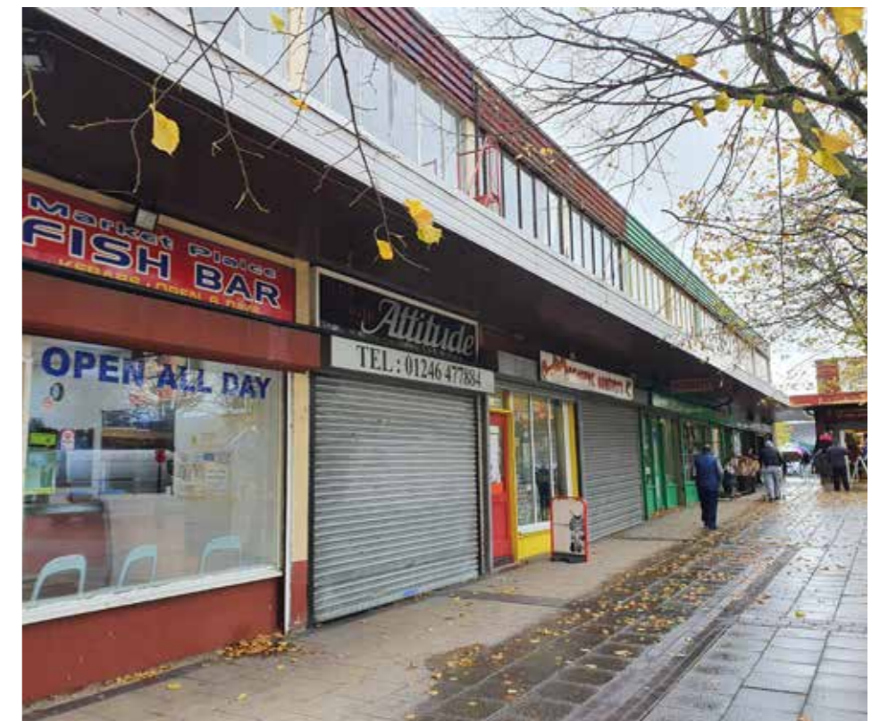
Market Square elevation of retail units.
