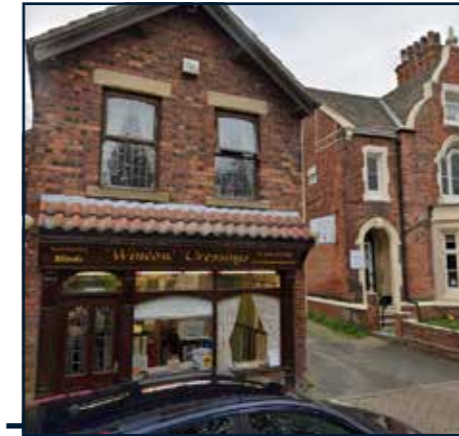
The north end of High Street shows off the red brick aesthetic of Staveley.
