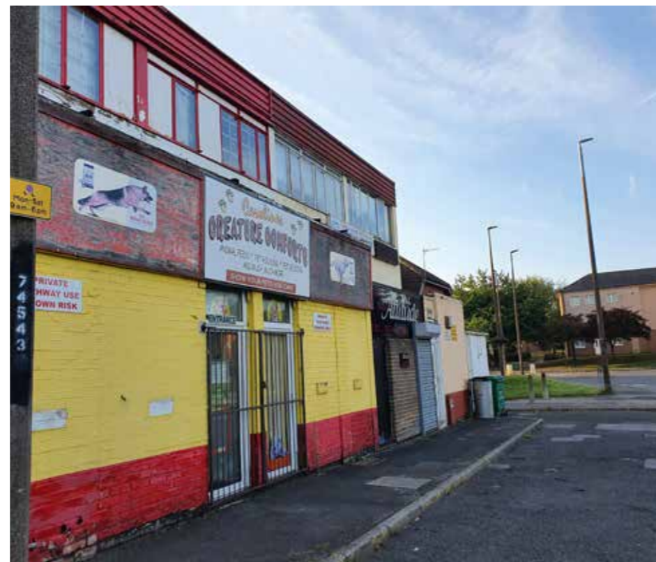
Barnfield Close elevation of retail units.
