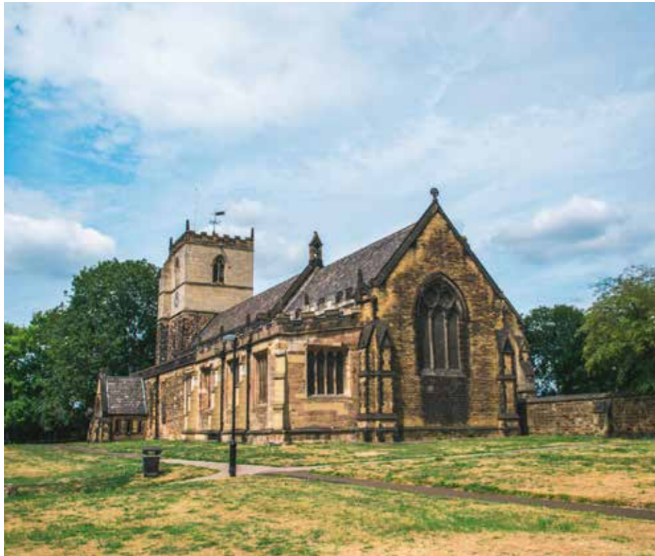
St John the Baptist Church, Church Street.
