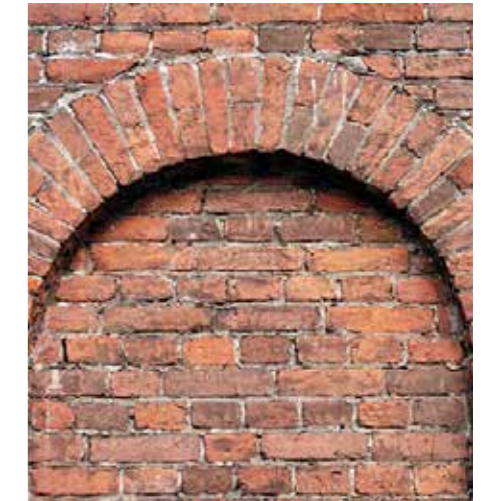
Soldier Course- Brickwork over the arch
