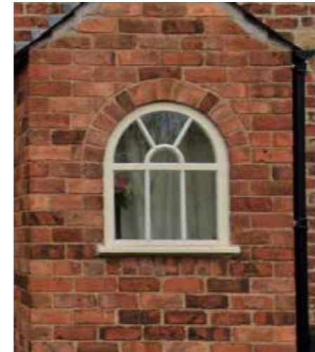
Existing Red Brickwork example in Staveley
